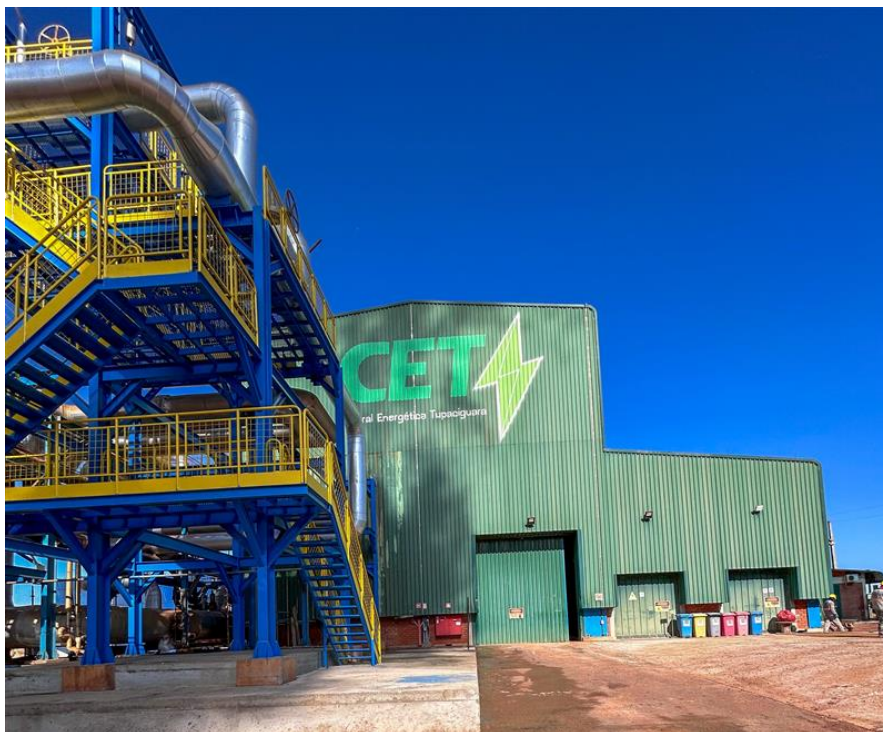
Thermal Generation Center
